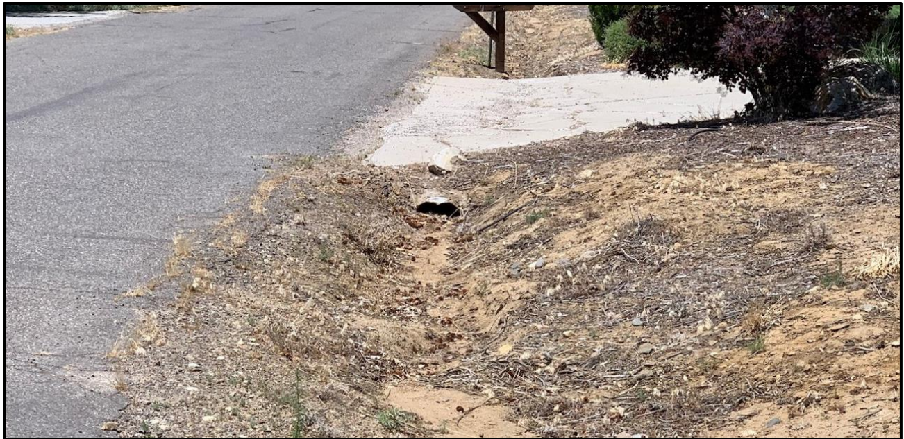
Figure 2-8. Example of driveway culvert in the study area with minimal capacity
