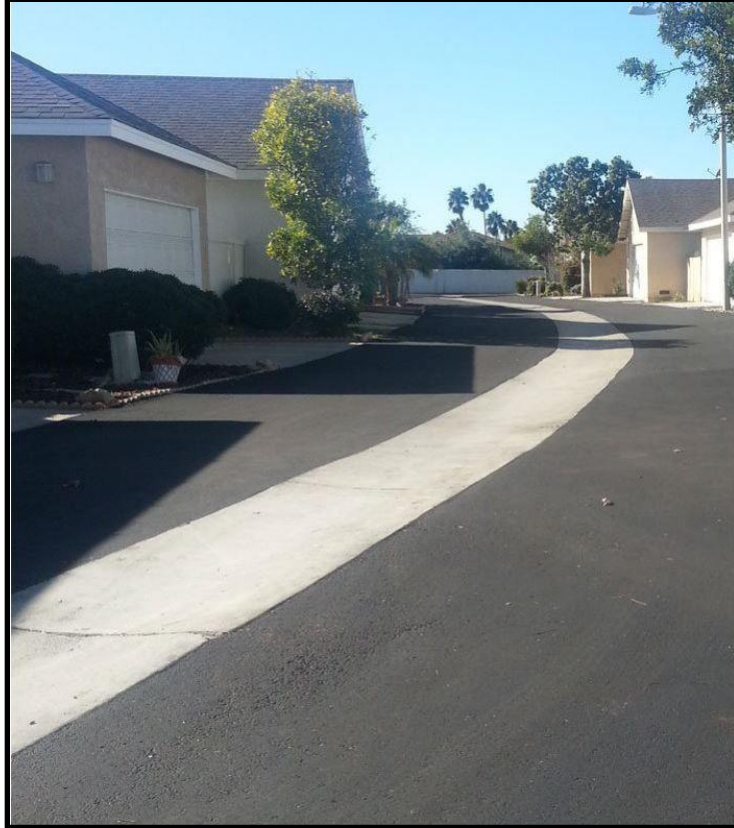
Figure 3-7. Example of a typical valley gutter
